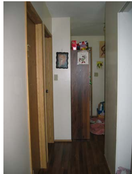
Hallways considered by some to be a waste of space; Kitsumkalum First Nation
