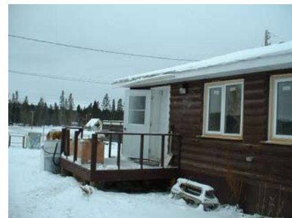
The need for an enclosed entrance, Liidlii Kue First Nation
