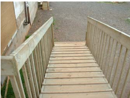
Entrance ramp, Naskapi Nation, Kawawachikamach
